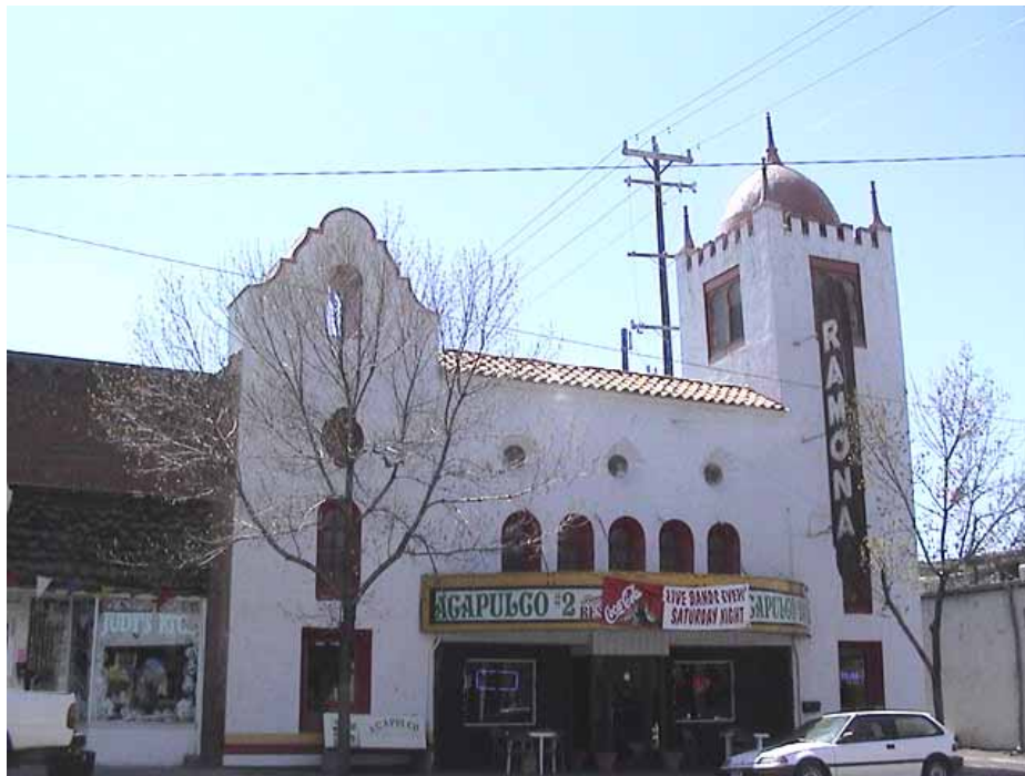
Buhl's Ramona Theater, which opened in 1928, seated 700 and could once again serve as a cultural hub for the community through historic preservation support from the Idaho Commission on the Arts or Idaho Heritage Trust.
